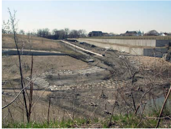
--Under construction April 2009
